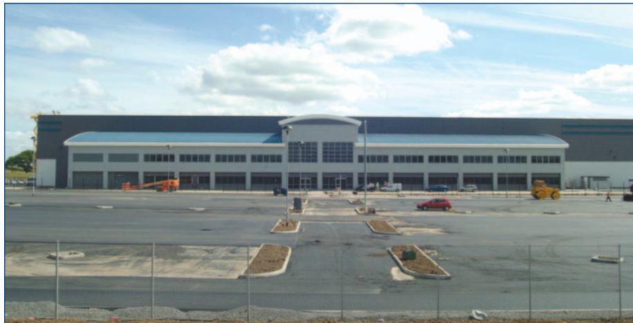
Argos Direct Regional Distribution Centre - nearing completion
