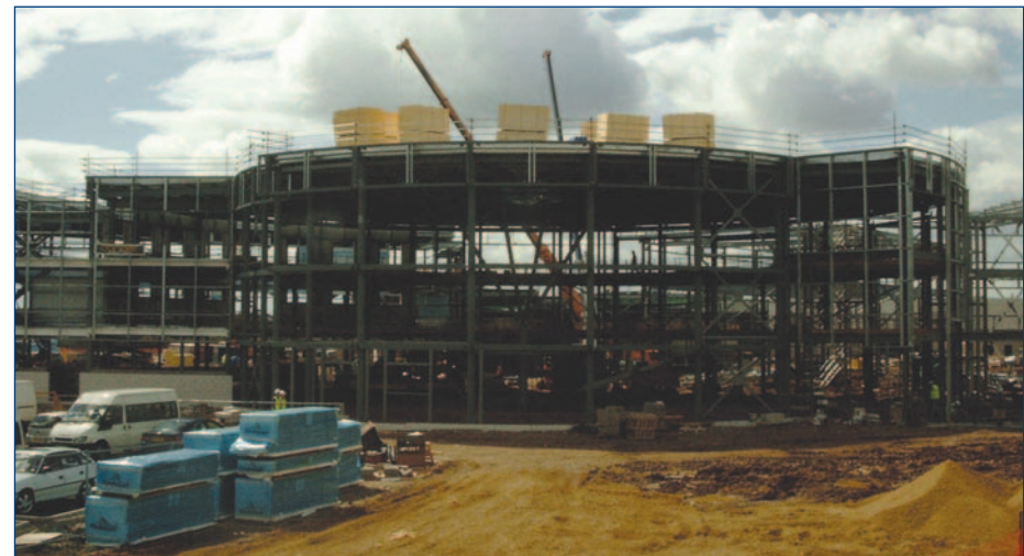
Construction of new Darlington College at Central Park
