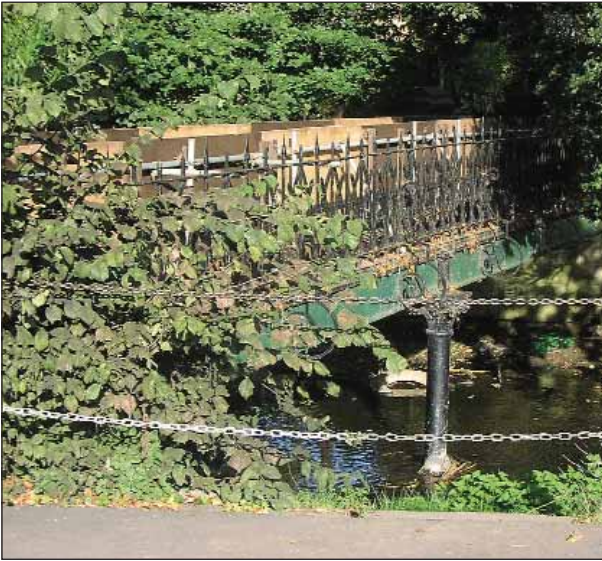
The cast and wrought iron and mild steel Polam Bridge, c.1890.
