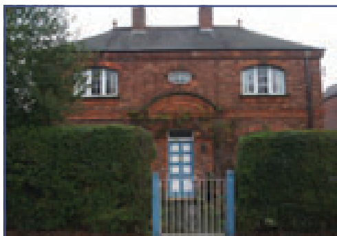
No. 8 Middleton Lane (former Edwardian police house)
