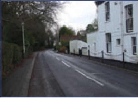
View eastwards along Church Lane
