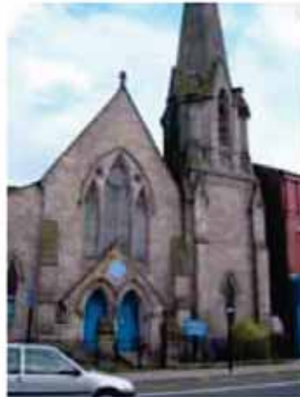
9. Grade II listed United Reformed Church, Northgate, constructed of locally-quarried stone from Houghton Bank (24)
