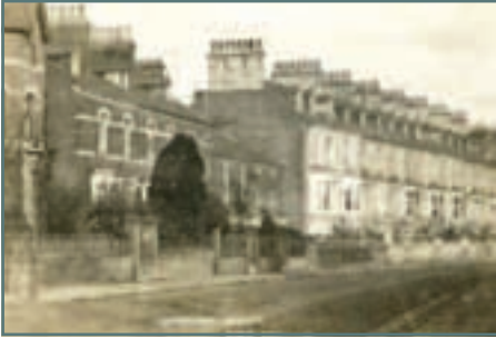
Pierremont Crescent, date unknown.
