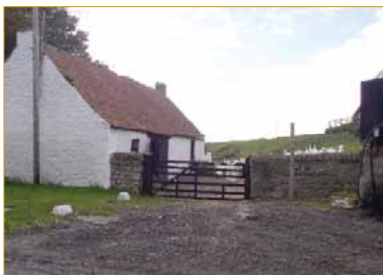
The cottage, South of Denton Hall cottages, identified as probably of 17th or early 18th date by its high pitched roof. Possibly originally thatched.
