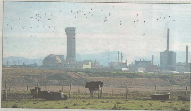
CONTRACT: Opentree, alongside Atlas Cloud, is helping bosses at Sellafield improve document management
