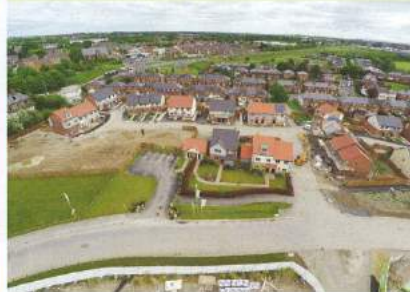
Work progressing on the Central Park development in Darlington
