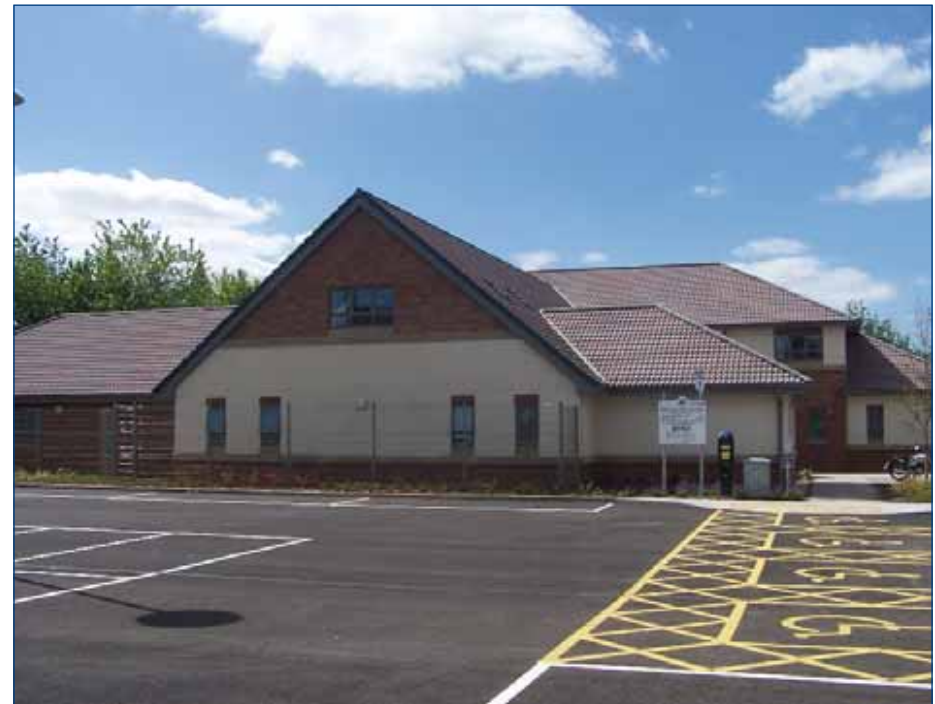
Park Place 'Secured Status' Car Park
