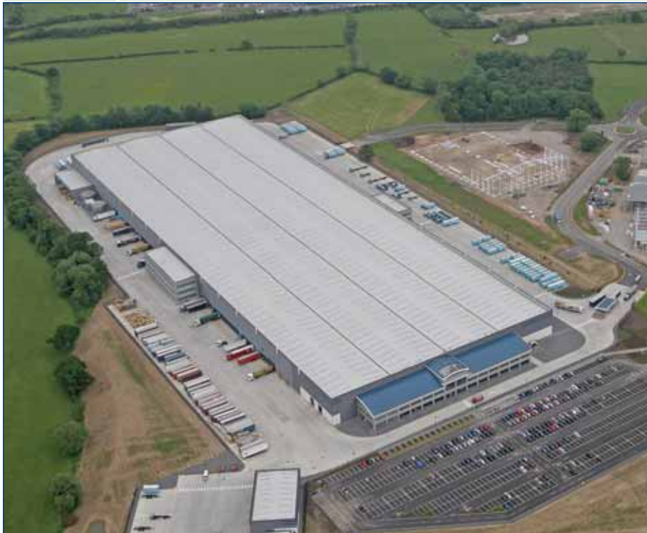
The completed Argos Direct Regional Distribution Centre
