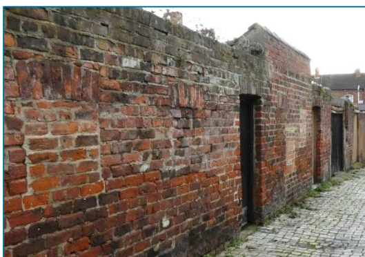
Left: Scoria-paved back lane off McNay Street lined by original rear-yard walling with openings, the coal holes now blocked. Right: Original metal railings in front of basements along Station Road. (Photos © Gaby Rose, 2023)
