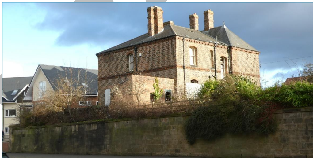
Top: Semi-detached houses possibly dating from the 1930s, with unusual front extensions. Centre: The terrace of former railway housing appears little altered. The modern building to the right is of no interest. Note the former higher road level. Bottom: Vicarage to St James church now derelict with tall retaining wall due to former lower road levels. Incongruous modern development in its immediate surroundings. (Photos © Gaby Rose, 2024)
