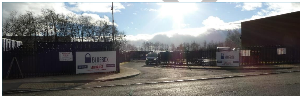
View from Cleveland Street onto the former site of Albert Hill Junction; many of the sidings would have stopped short of the road, although others did cross it to serve the Darlington Forge. (Photo © Gaby Rose, 2024)
