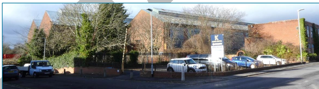
Top left: Stone-and-metal railway bridge over Elmtree Street, west elevation. Top right: Former Alexandra Hotel, now the St Georges Bridge Centre. Middle: Prominent buildings and retaining wall of Rise Carr Rolling Mills site along Whessoe Road. Bottom: Level car park and Prospect Way (left) at entrance to Rolling Mills site. (Photos © Gaby Rose, 2024 & 2023 for top right only)
