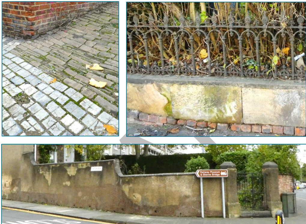
Top left: Back lane with scoria and sandstone block surfacing. The scoria bricks were produced (possibly from 1899) by the Tees Scoria Brick Co. Ltd of Bank Top, Darlington, and were the by-product of the steelmaking industry in Middlesbrough. Their high mineral content resulted in the distinct blue colouring. Designed to combat disease-ridden back alleys, these bricks were easily washable. Top right: Ornate, cast-iron railings on ashlar stone/brick boundary walling between private front garden and public realm. Bottom: Rendered garden wall on street corner with stone copings and prominent gate piers; also note the poorly placed signage (Photos © Gaby Rose, 2023)
