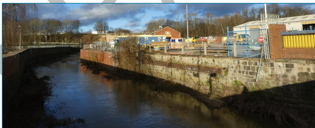
Top: Stepped brick walling with recessed panels along south (John Street) and east boundaries of the commercial site. Bottom: View from John Street Bridge onto proposed extension area including traditional brick building in the background; [7] Skerne Bridge can just be glimpsed to the left of it. (Photos © Gaby Rose, 2024)
