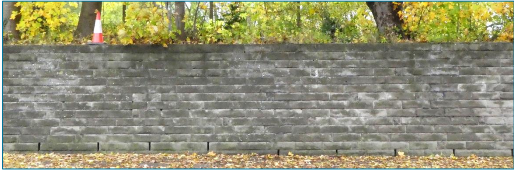
Coursed sandstone retaining wall along Hopetown Lane enclosing railway site with mature vegetation behind (Photo © Gaby Rose, 2023)
