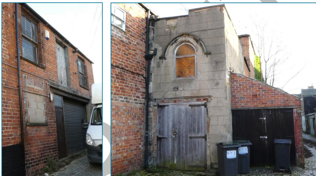
Left: Outbuilding with hoisting door. Right: Various brick and rendered outbuildings along the longer back lane, the central one being Tallyman's Cabin, which used to be crenelated and has a Neo-Gothic entrance behind the abutting brick garage (Photos © Gaby Rose, 2023)
