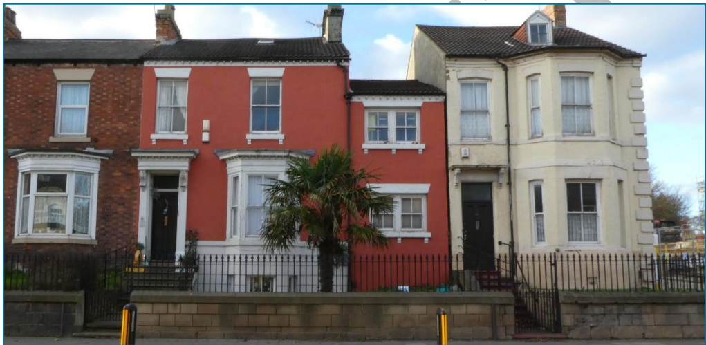
Top: No.s 105 (grey) and 109 (end property) High Northgate prior to works. No. 105 including its boundary wall was improved under the 2002-05 HERS, and No. 105 under the 2005-09 PSCA, including new metal railings. (Photo © DBC, before July 2001). Bottom: The properties are still standing out positively today. (Photo © Gaby Rose, 2023).
