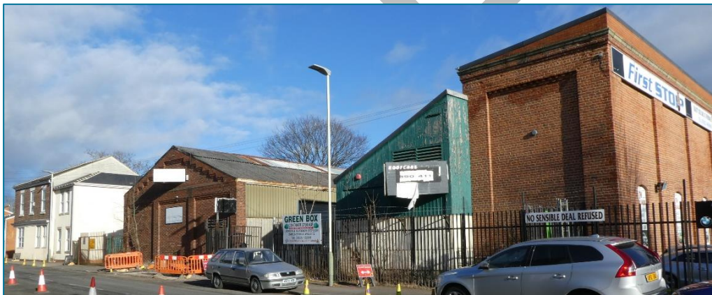
Top: The former Globe pub, now flats; the attached building is modern. Bottom: The former water tower is the brick building on the right, the tank now removed and a new roof provided. Attached to it is one of the timber structures shown on the 1939 map. The brick building on the left marks the northwest corner of the former Locomotive Works and, like the water tower, has recessed panelled brick walling. (Photos © Gaby Rose, 2024)
