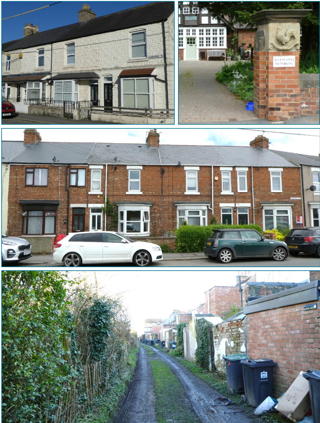
Subzone D1: Top left: Harpers Terrace faced in cast stone, with shallow front gardens. Later canopies spanning between bay windows cut into and obscure the decorative string courses at Nos. 1-4. Whilst the window frames have been changed to different designs, the opening pattern has been well preserved. The decorative lintel design to Nos. 1 and 2 (right) can also be found on window openings to the rear of Station Terrace (Photo © Gaby Rose, February 2025). Top right: Entrance pier with carved stone cockerel, which was brought here from Low Middleton Hall 175 , and two commemoration plaques on the gable wall in the background, [M] Cocks Memorial Homes. Middle: The long Station Terrace with three well preserved houses, although window frames have been changed to different designs. The unit on the left, which would have looked the same, has been changed significantly, like many other houses in this row (Photos © Gaby Rose, May 2024). Bottom: Back lane to rear of Station Terrace with overgrown former allotment gardens to the left/east. (Photo © Gaby Rose, February 2025)
