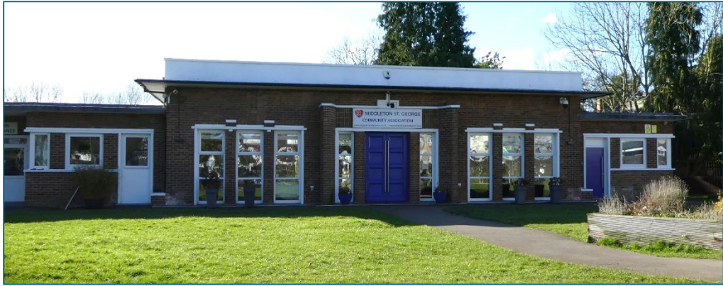
Former [L] Pumping Station, now Community Centre, built in a Modernist style. The original multi-pane windows have been replaced. (Photo © Gaby Rose, February 2025)
