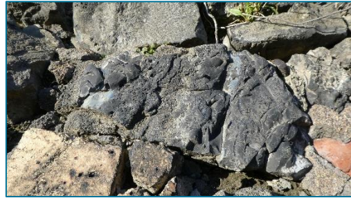
Top: Remains of southern boundary wall of the [Q] Middleton Iron Works, bordering the back lane to Killinghall Row, Yarm Road, the first houses to be built for the increasing workforce. It is mainly constructed from slag with a few red brick pinnings in between. Smelting is the process of applying heat and a chemical reducing agent to an ore to extract a desired base metal product. As most ores are impure, it was necessary to use limestone, which was brought in from Weardale, to remove the accompanying rock gangue as slag 101 . This wall is now the only survivor of the iron works site (Photo © Gaby Rose, March 2024). Bottom: Details of slag pieces. (Photos © Gaby Rose, February 2025)
