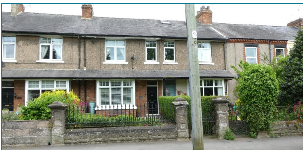
Water View, the southern terrace, of which parts have been rendered. There is a continuous ground-floor canopy and the original opening pattern has been preserved. The front garden in the middle has an unusual stone boundary wall with metal railings and distinct carved piers, which are in poor condition. Note the eaves detailing on the right-hand, earlier house. (Photo © Gaby Rose, May 2024)
