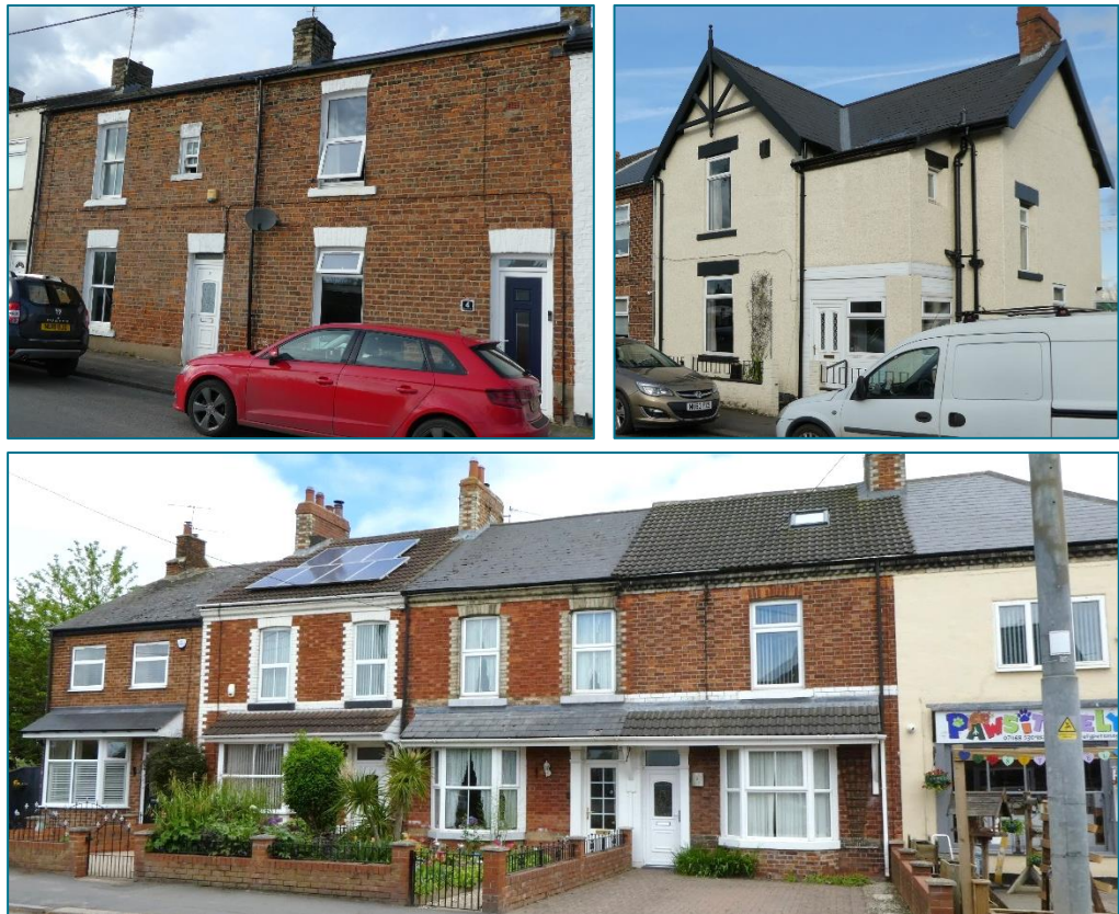
Subzone D2: Top left: Two well-preserved houses at Killinghall Row, the first terrace built for the iron workers, which face directly onto the pavement. Top right: Former stationmaster's house for Dinsdale Station at the south end of Belle Vue Terrace (Photos © Gaby Rose, March 2024). Bottom: Harts Buildings at the southern end of Station Road with polychromatic brickwork. Whilst Nos. 1-4 appear to be built around the same time, there is a clear change in construction between Nos. 2 and 3, including different eaves and window surround designs, and the use of a different type of red brick. The once continuous roof surface has now been broken up by using different materials. (Photo © Gaby Rose, May 2024)
