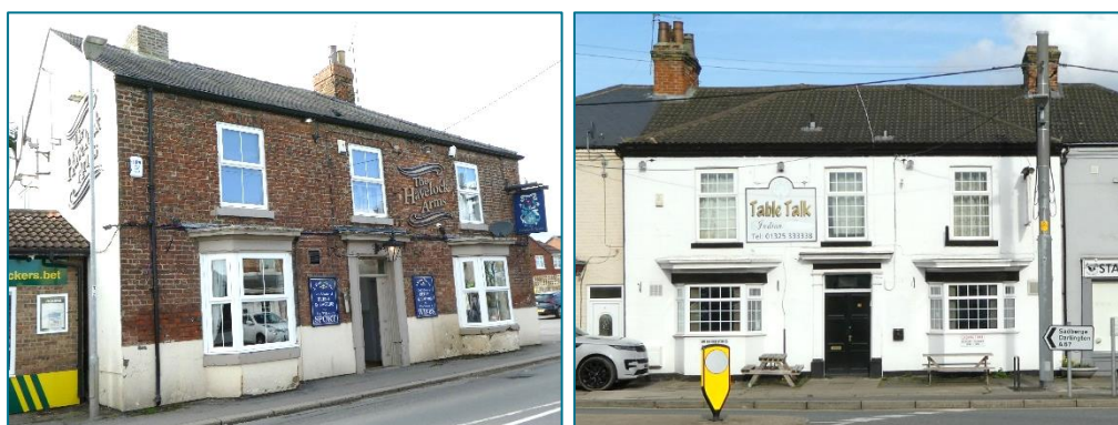
Left: [N] Havelock Arms Hotel. Right: The former [O] Killinghall Arms; a historical photo shows the building without render and 2x2 sliding sashes 110 . (Photos © Gaby Rose, March 2024)
