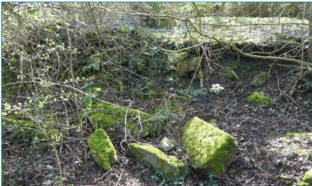
[A] Crane Base (top) and Platform (bottom). Top : Looking northwest, the platform is behind the crane base within the undergrowth; its alignment shown on the 1913 map is indicated by the yellow line. The rail tracks coming from the main railway line would have been to the righthand/northeast side. Bottom : Remnants of former platform viewed from the bridlepath looking southwest, with the walling stones now largely dislodged. The crane base is to the left/south just outside the view. (Photos © Gaby Rose, March 2024)
