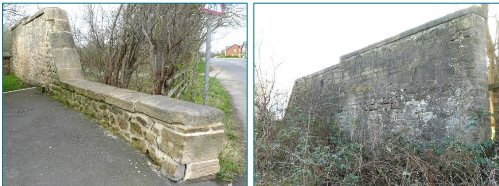
Remains of possibly original (1825) boundary walling of the [D] Coal Depot constructed in squared sandstone. Left: View looking north with Sadberge Road to the right. The end of the wall has been damaged, possibly by a wagon 70 . Right: View from the disused railway corridor looking south. (Photos © Gaby Rose, March 2024)
