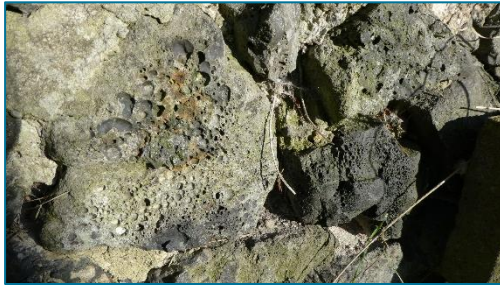
Top: Remains of southern boundary wall of the [Q] Middleton Iron Works, bordering the back lane to Killinghall Row, Yarm Road, the first houses to be built for the increasing workforce. It is mainly constructed from slag with a few red brick pinnings in between. Smelting is the process of applying heat and a chemical reducing agent to an ore to extract a desired base metal product. As most ores are impure, it was necessary to use limestone, which was brought in from Weardale, to remove the accompanying rock gangue as slag 101 . This wall is now the only survivor of the iron works site (Photo © Gaby Rose, March 2024). Bottom: Details of slag pieces. (Photos © Gaby Rose, February 2025)
