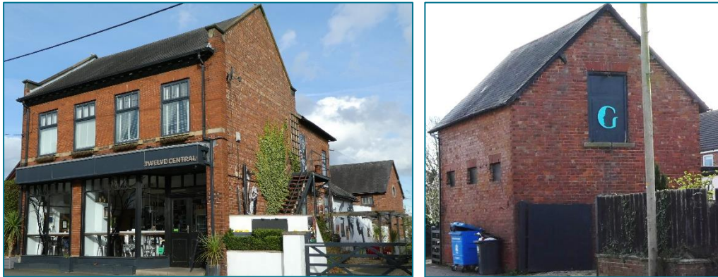
Left: Former [P] Co-op along Middleton Lane with detached Stable building in the background. Right: Stable viewed from Yarm Road. (Photos © Gaby Rose, March 2024)
